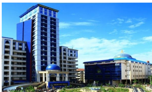
Figure 2 Iqra' Tower Building Unismuh Makassar
