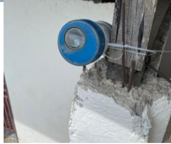
Figure 2. Installation of the SQM with housing at the mosque in Sungai Rumpun Village.
