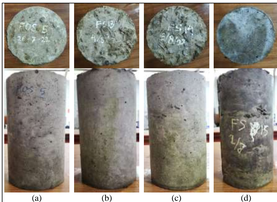
Figure 2. Visuals appearance of concrete sample due to salt attack for 56 days soaking, which is the CF content: (a) 0%; (b) 0.3%; (c) 0.5%; (d) 1.0%
