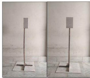
Figure 7. Implementation of Long Range RFID Box Construction
