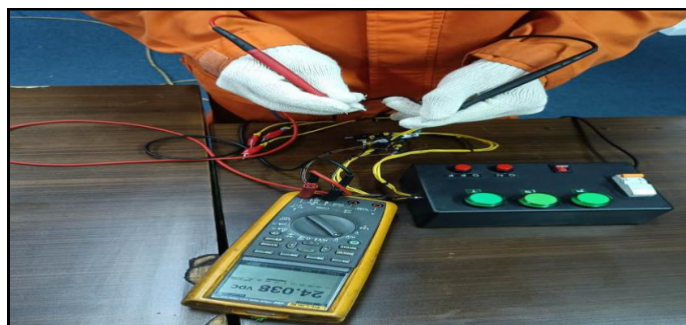
Figure 6. DC Output Voltage Testing
