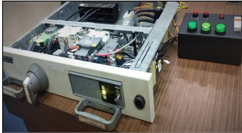
Figure 12. Testing the OFF indication on a 3 Phase 380 V CB
