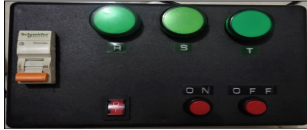
Figure 11. Testing CB Output 3 Phase 380 V Order OFF
